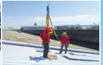
KS Reroof & Renovate
